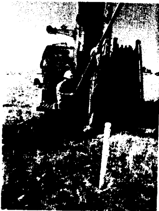
39. Installing inclinometer, piezometer in foreground (... 071002 to 05 Field Trip 045.jpg
