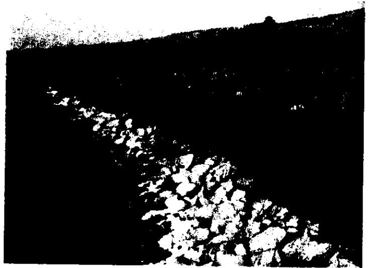
2. West from point, good rip rap armour 071002 to 05 Field Trip 008.jpg
